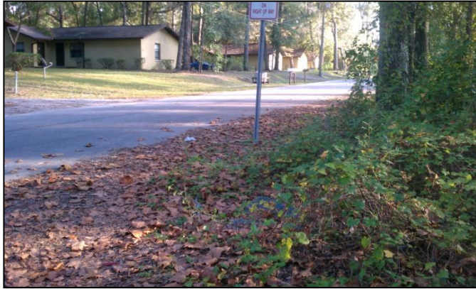
This photograph was taken from the West side of the road, at NE 56th Ave. No sidewalks, gutters, curbs, stormwater.
