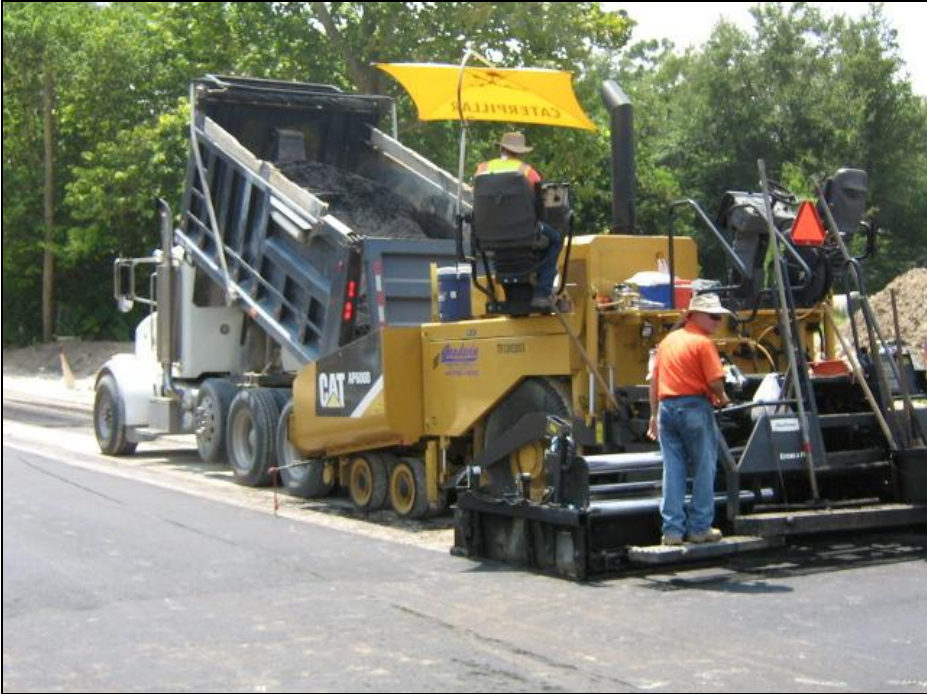
Placing asphalt on the NW 35 th Street, Phase 1B project.
