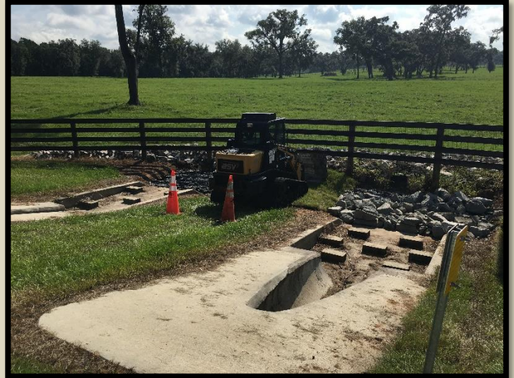
Erosion repair at end of pipe
