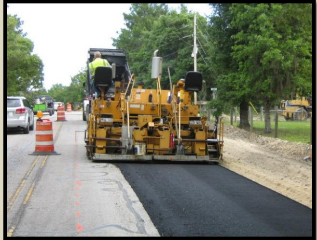
County Road 314A rehabilitation project
