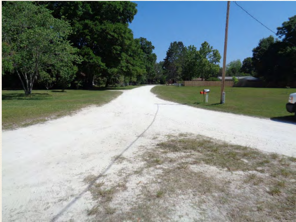
Northeast 17th Court looking north from Northeast 90th Place
