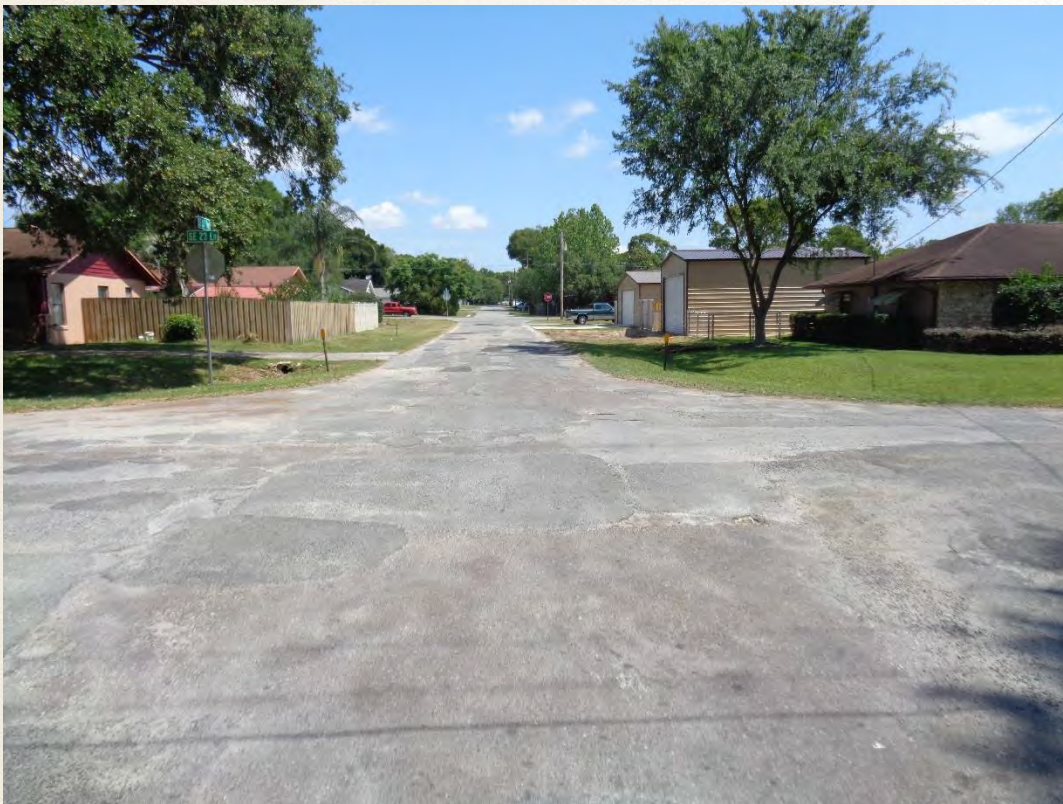
Southeast 56th Terrace looking north from Southeast 23rd Lane
