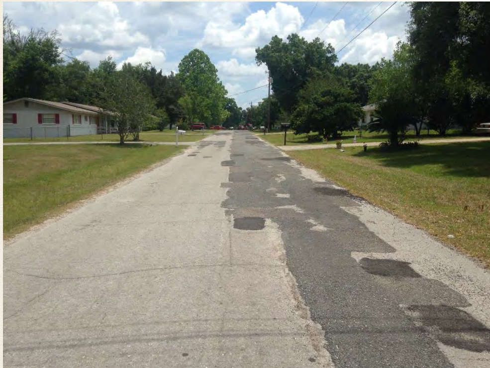
Northeast 50th Street looking east from Northeast 18th Court
