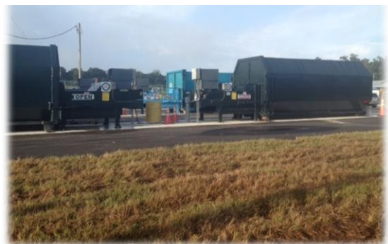
View of Garbage and Recycle Compactors
